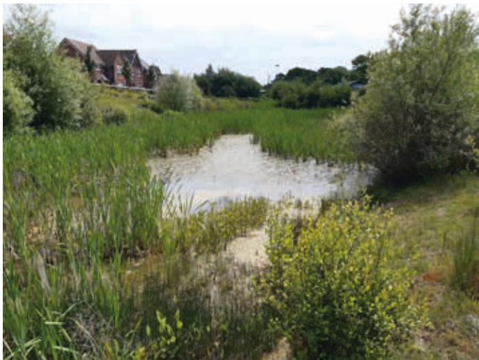
Gallows Cross SuDS pond 2022: Within two years the beds of Reedmace and Reeds had almost eliminated open water
