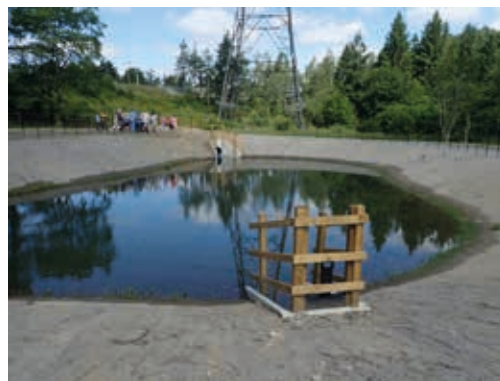
Stover South Sedimentation Pond 2019: one of Stover's primary sedimentation ponds after completion in 2019.
