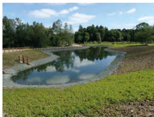
Stover South Balancing Pond 2019: One of the 'reedbed' filtration ponds at Stover after completion in 2019.
